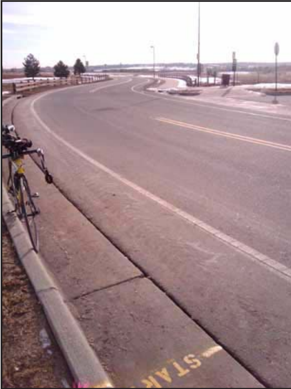
Start, looking east
