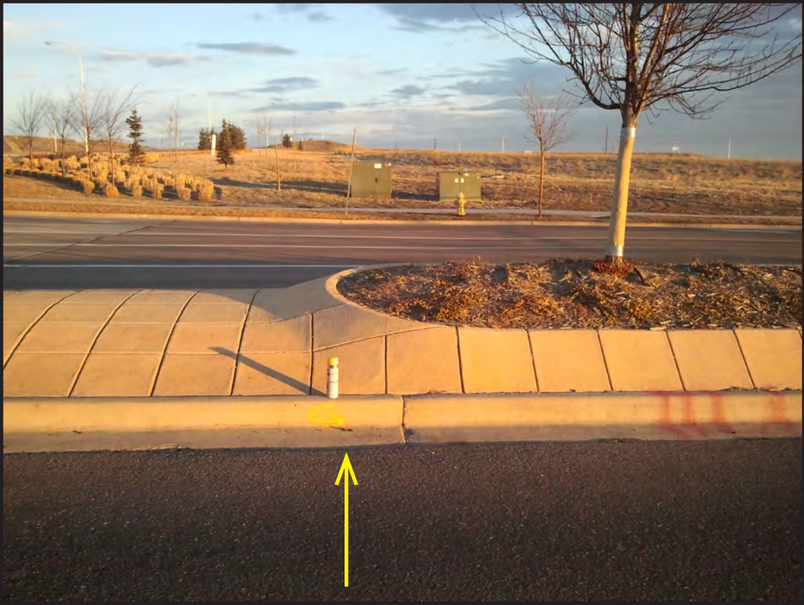
Turnaround, looking north
