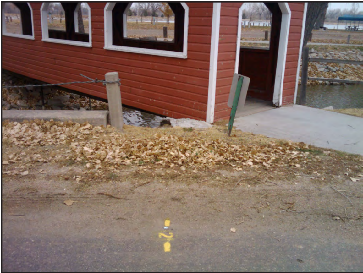
2k Start, looking north
